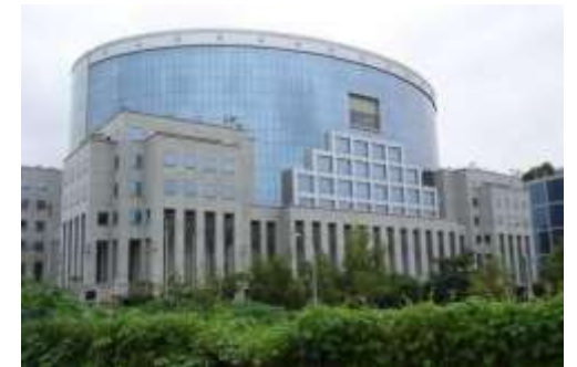
MMRDA HQ, Mumbai, India
