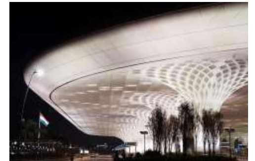
Mumbai Airport, India
