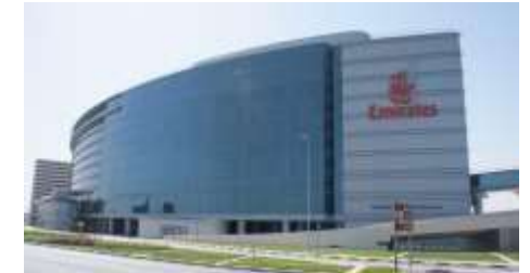
Emirates Airlines HQ, Dubai
